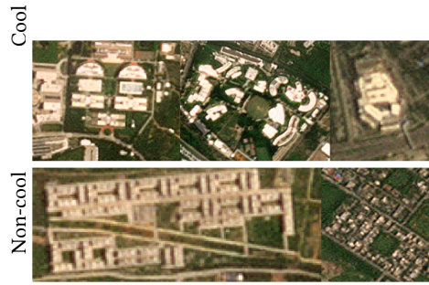
Fig. 5. Visual validation of our dataset, where the top row showcases regions with cool roofs and the bottom row showcases regions with non-cool roofs. From left to right in the top row, buildings are located in Hyderabad, Tamil Nadu, and Noida. In the bottom row, from left to right, the locations are Hyderabad and Anand. Cool roofs should appear brighter compared to non-cool roofs
